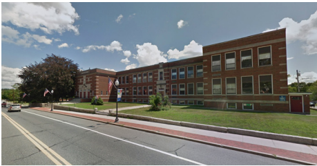
From the top: Construction underway at the former American Legion Building on West Central Street, the town-owned Middlesex Avenue parking lot and the Saint Patrick's property.
