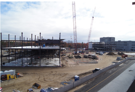
MathWorks New Lakeside Campus Under Construction.
