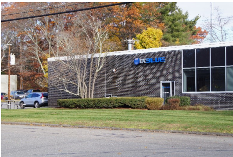
Erie Drive in the East Natick Industrial Park
