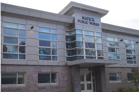
Public Works Building
